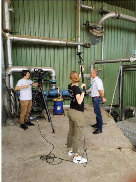
Figure 8: Shooting in front of the feeding system in Utzenaich (biogasplant, Austria)
