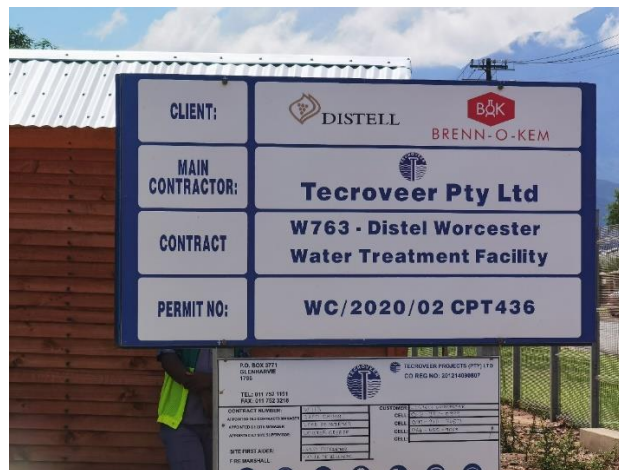
Figure 29: Distell & Brenn-O-Kem Water Treatment Facility
