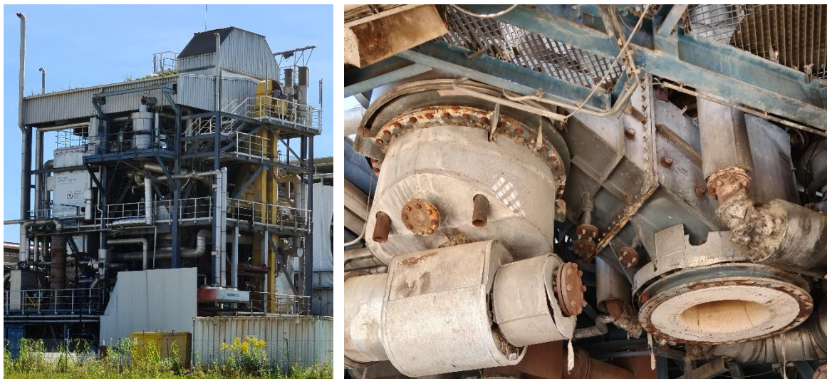
Picture 16: Fast Internally Circulating Fluidized Bed gasification plant in Güssing, Austria: left: whole plant; right: bottom of gasifier and autothermic bed recirculation chamber
