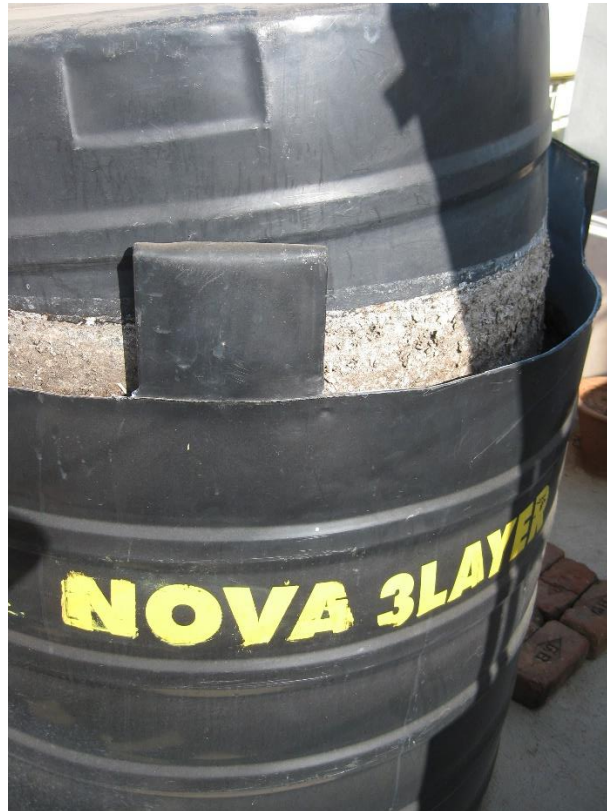
Picture 73: Gap between the inner and outer tube. Source: German Biogas Association
