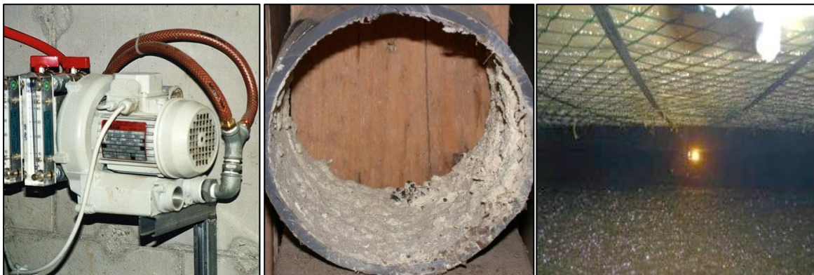
Picture 65: Left: blower for desulphuration with air, middle: elementary sulphur within a gas pipe, right: sulphur at the top of the digester.
