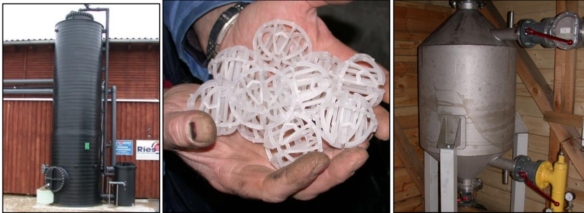
Picture 66: Left: external desulphurization column, middle: padding material for sulfobacter oxydans within external desulphurization column, right: activated coal filter.
