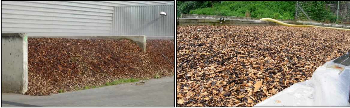
Picture 14: Biofilter filled with wood chip as bedding material for odour substance degrading bacteria.
