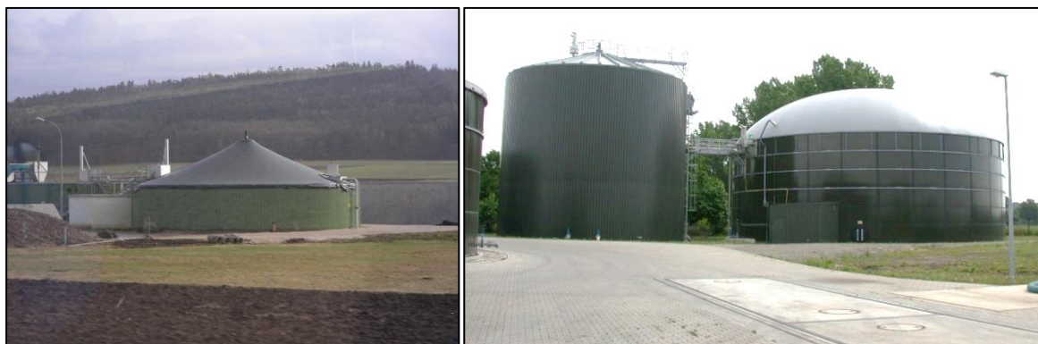
Picture 61: Left: double membrane with middle pole, right: digester with inner single membrane suspended from roof on the left and digester with double membrane shaped by air blower on the right.
