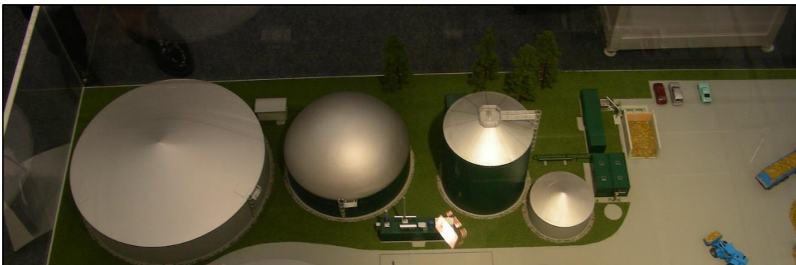
Picture 20: Model of a biogas plant with multistage digestion process (feeder, storage tank for slurry, main digester, post digester, gas-tight storage tank).
