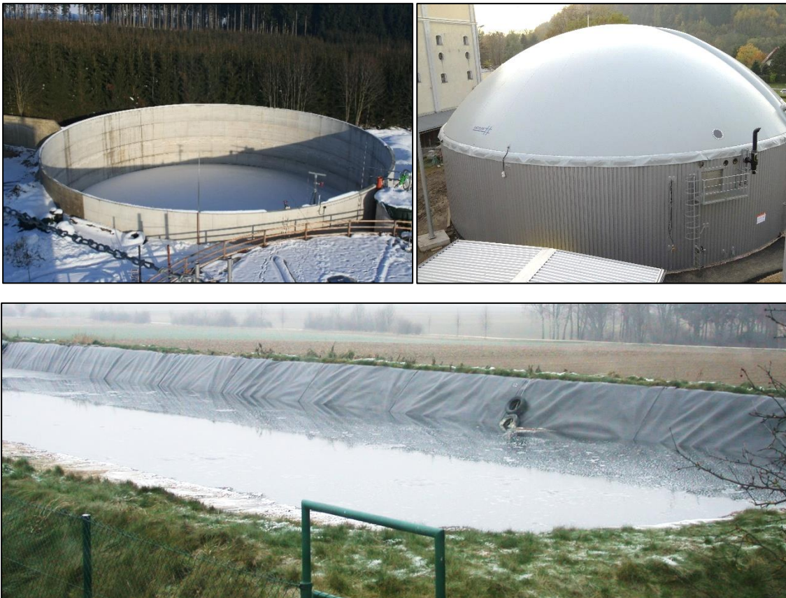
Picture 55: Digestate storage tank: top left: open storage tank, top right: airtight gas storage tank with a double membrane layer and connection to the gas system, below: open lagoon with double layer membrane to monitor tightness.
