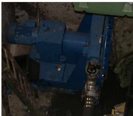
Picture 36: Peristaltic pump.
