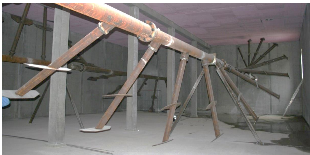
Picture 28: Slow speed agitator in a horizontal digester.
