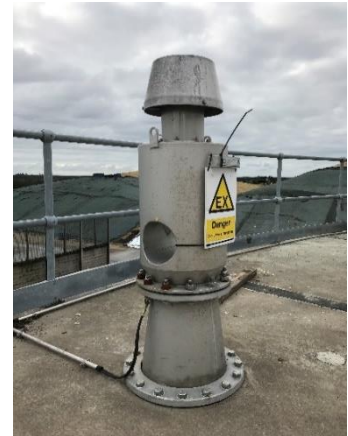
Picture 41: Over and under pressure valve. Important to notice that exhaust pipe must be outside.
