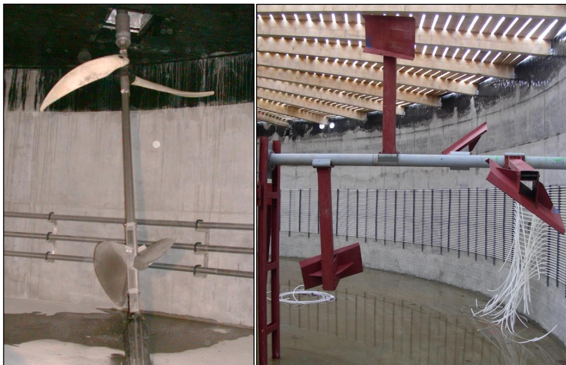
Picture 27: Different types of slow speed agitators.
