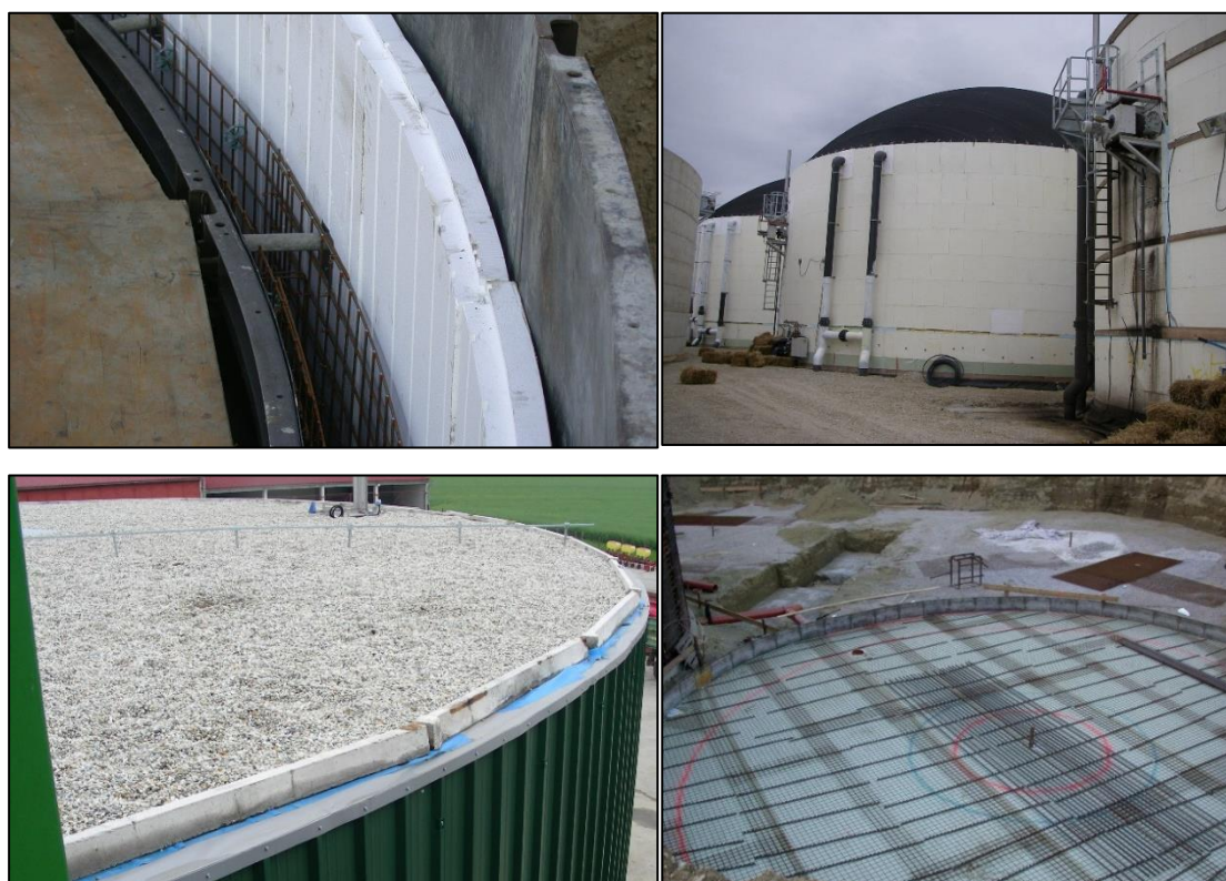
Picture 24: Types of wall isolation, top left: special confectioned isolation which is included in the process of casting the concrete, top right: isolation outside of digester through nails, bottom left: sandwich panels, bottom right: isolation under the floor.
