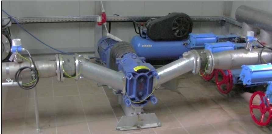
Picture 47: Pumping station with pressure sensor before and after the pump to detect distortions.
