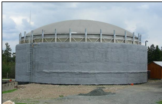
Picture 63: Wet gasometer directly included in the digester storage tank.
