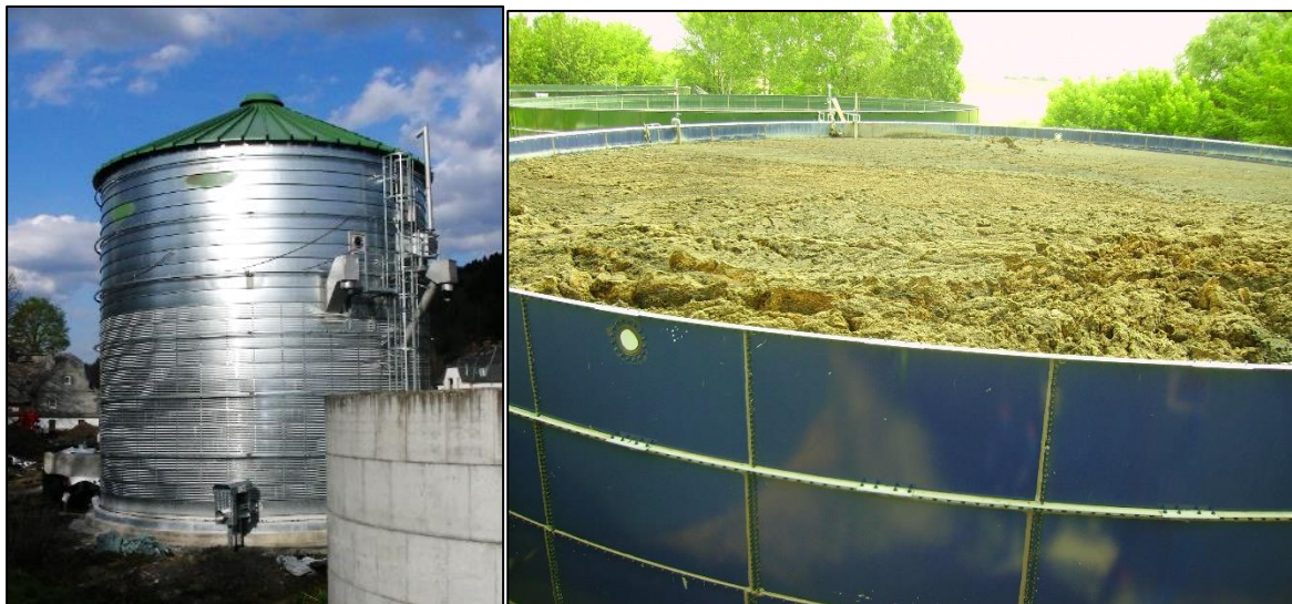
Picture 23: Digester material: left: rolled stainless steel digester with floor heating pipes on the outside, right: enamelled steel storage.
