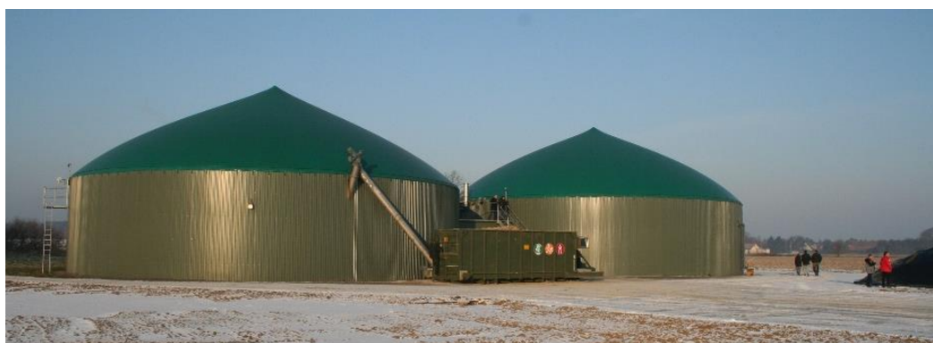
Picture 21: Typical biogas plant with a main digester followed by a post digester.
