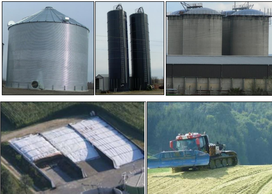
Picture 2: Different types of storage systems: top left: not gas-tight silo, top middle: gas-tight silo where conservation is done with carbon dioxide, top right: air-tight silo where conservation is done through lowering pH value, bottom: air-tight clamp silo, where compression is done with heavy machinery like tractors or even snow groomers.
