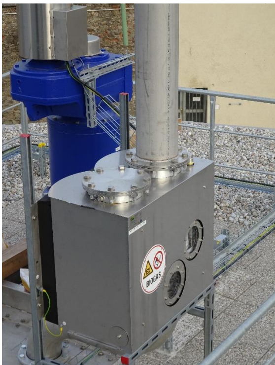
Picture 42: types of over and under pressure valves, Important to notice: no valve has to be installed between valve and digester, exhaust pipe has to be outside of contact area, if installed outside it needs to be secured from freezing.
