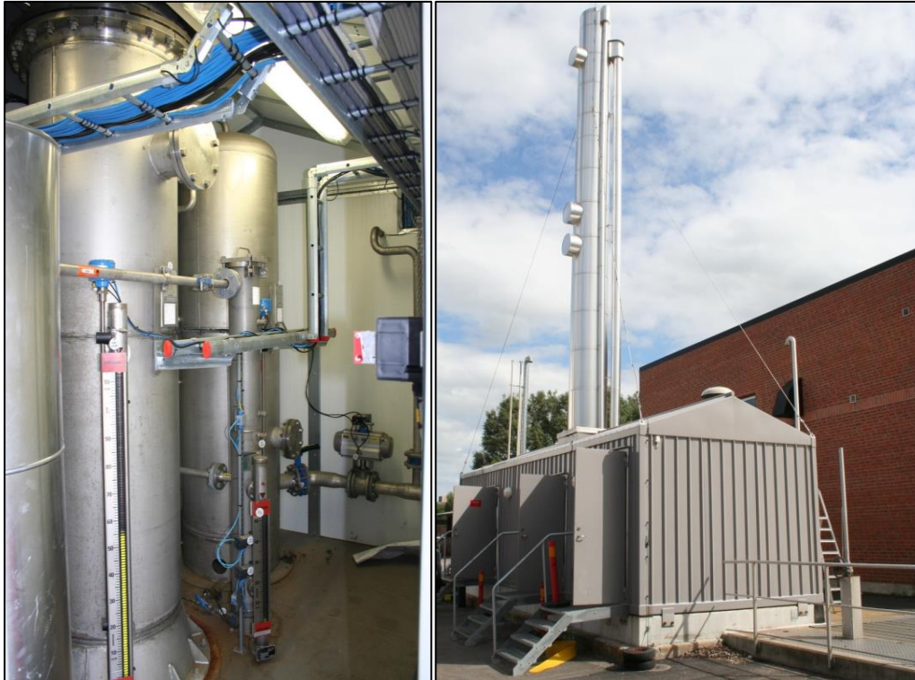
Picture 70: CO 2 separation through water scrubber left: scrubber column, right: water scrubber technique installed in a container.
