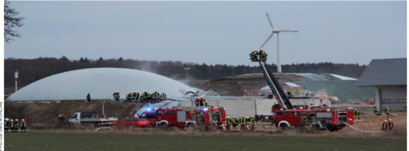
Source: Biogas Safety first! Guidelines for the safe use of biogas technology; Fachverband Biogas e.V.; Photo: Uwe Mühling
