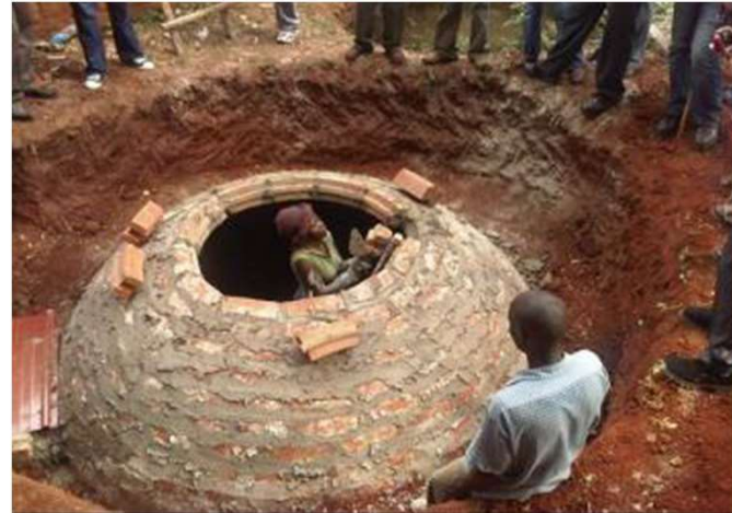
In-situ cast Puxin Digester
